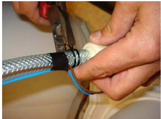
Assemble hose clamps
